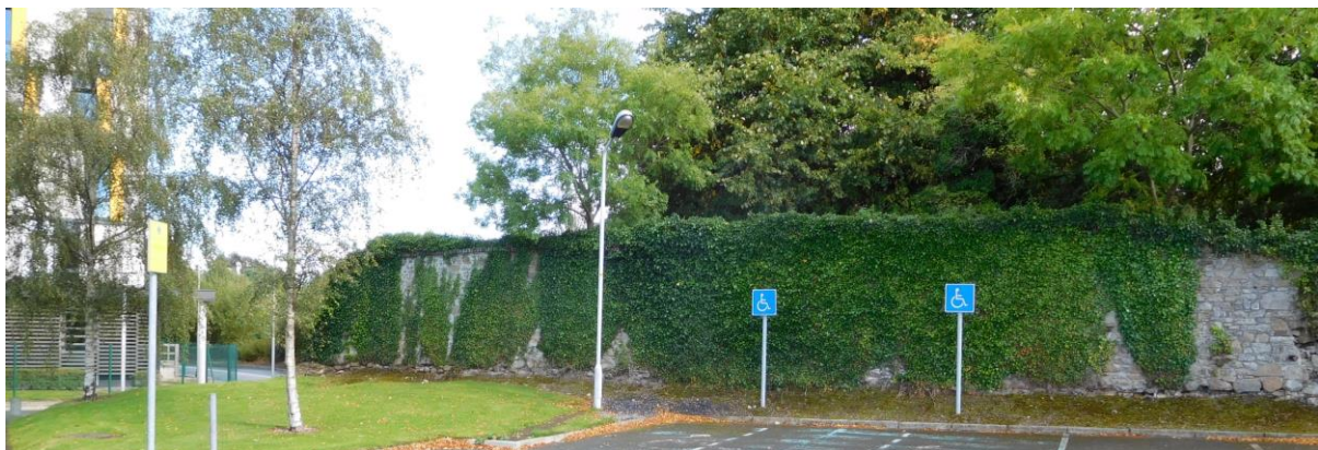
Figure 15.19 Northern Corner of Stone Wall
