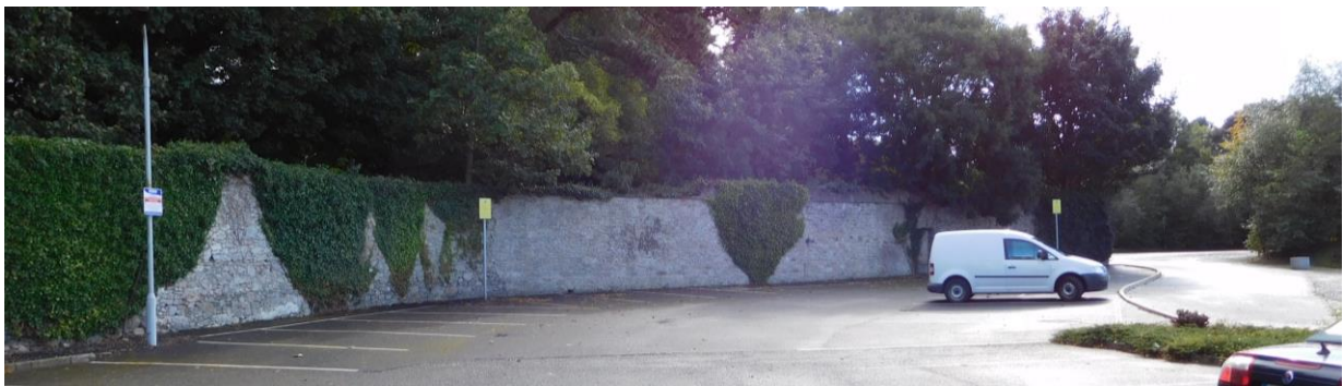
Figure 15.21 End of Northern Section of Stone Wall
