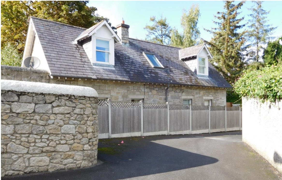
Figure 15.26 East Façade of the Glebe Lodge
