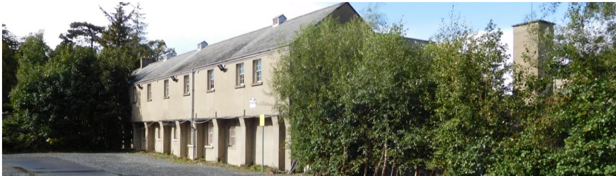
Figure 15.15 View of the Courtyard to the South of the Church, looking North
