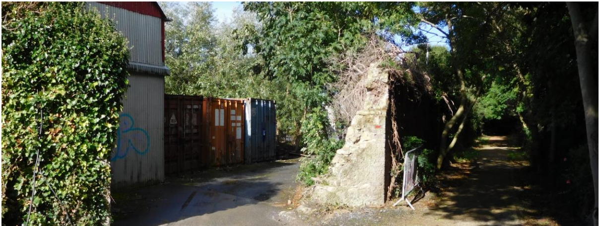
Figure 15.24 Southern Corner of Stone Wall, near the Crannog Lodge
