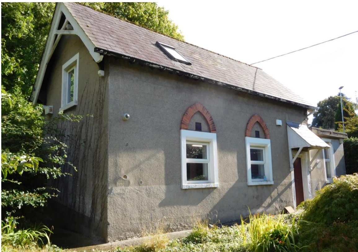
Figure 15.29 Part View of the Western and Southern façades of the Crannog Lodge
