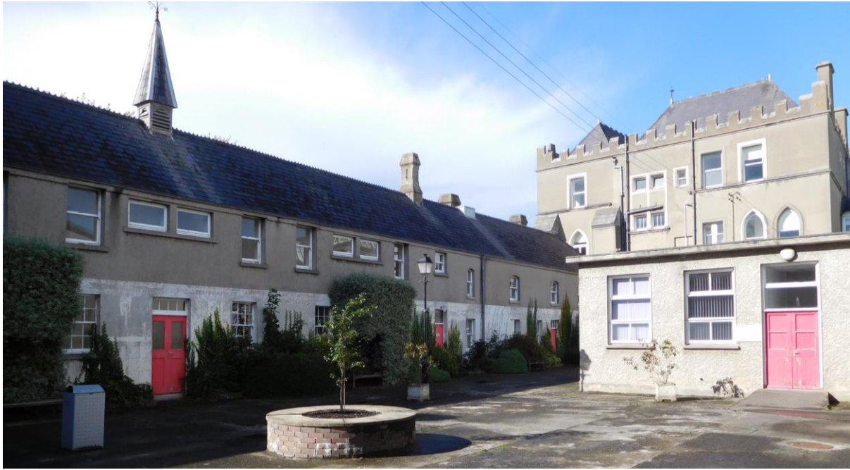
Figure 15.11 Southern Façade of Roebuck Castle, viewed from first courtyard, looking towards church
