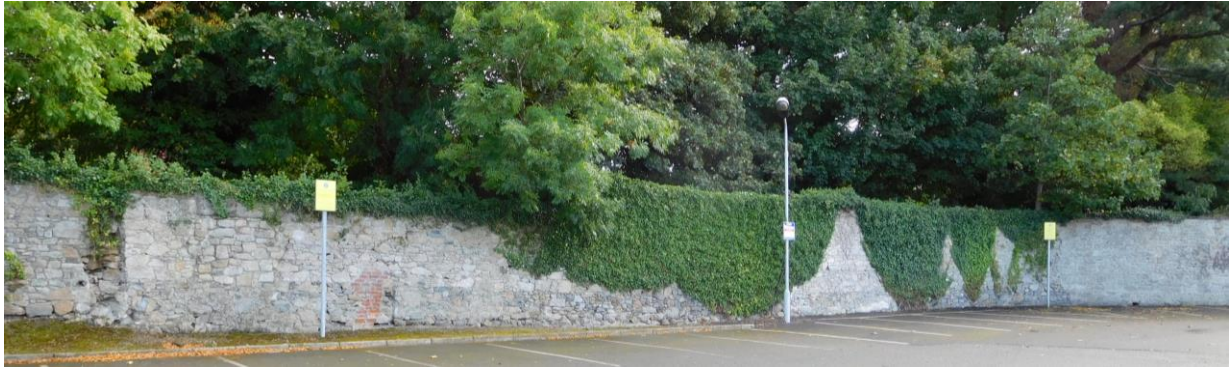
Figure 15.20 Continuation of Northern Part of Stone Wall
